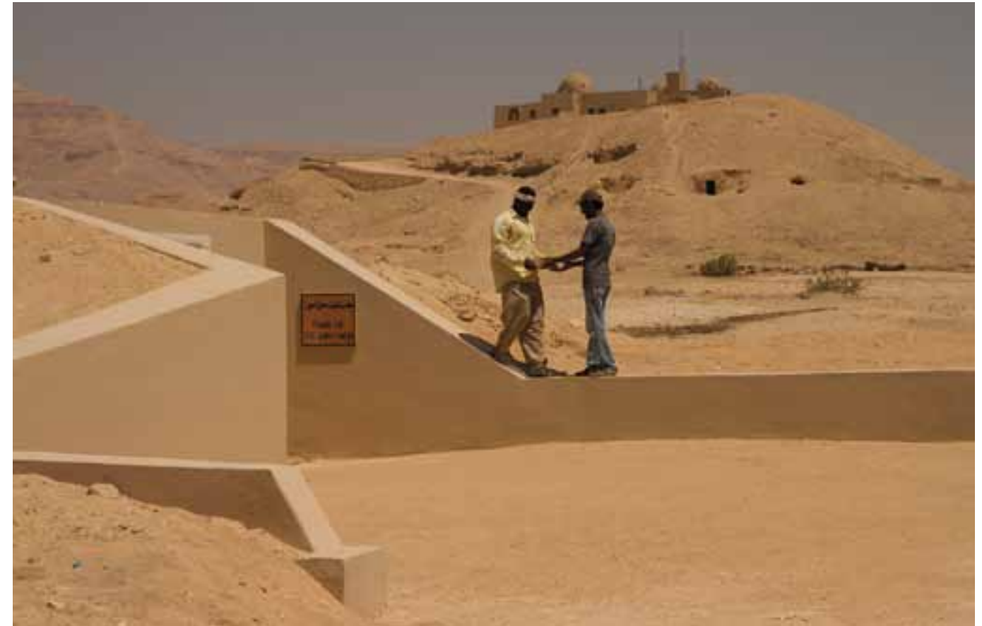
The entrance to the facsimile of the tomb of Tutankhamun with Stoppelaere house in the distance.
