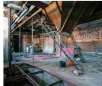
The condition of the Silo building when purchased in 2020
