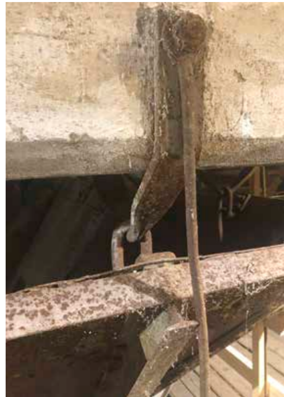
Flexible 'organic' metal joints - to be repurposed as part of a balustrade system
