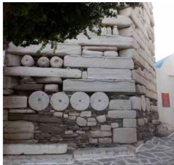
The Frankish Castle of Paros, Parikia Island: Built by Venetians in the 1200s from the remains of ancient sanctuaries
