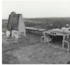
Demolition of the Toppila Ltd Factory in 1993, Kaleva Archives
