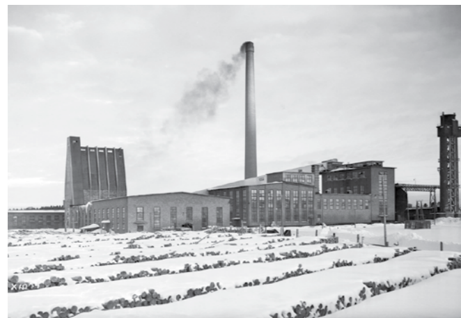
Toppila Pulp Mill shortly after completion (1930's), snow covered wood in the foreground. Finnish Heritage Agency
