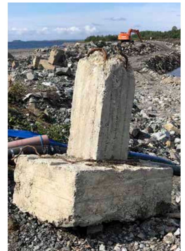
Concrete waste used as landfill for the new marina in Meri-Toppila, Oulu
