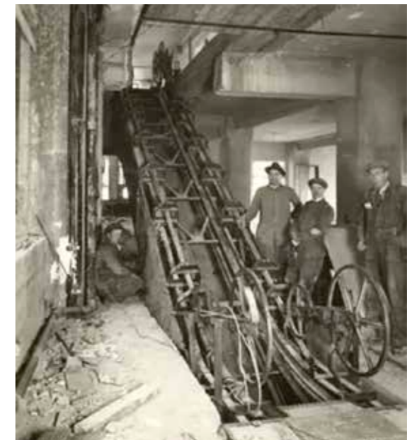
One of KONE's industrial conveyors, 1930, of the same type used in the AaltoSiilo and Toppila Pulp Mill in 1931.
