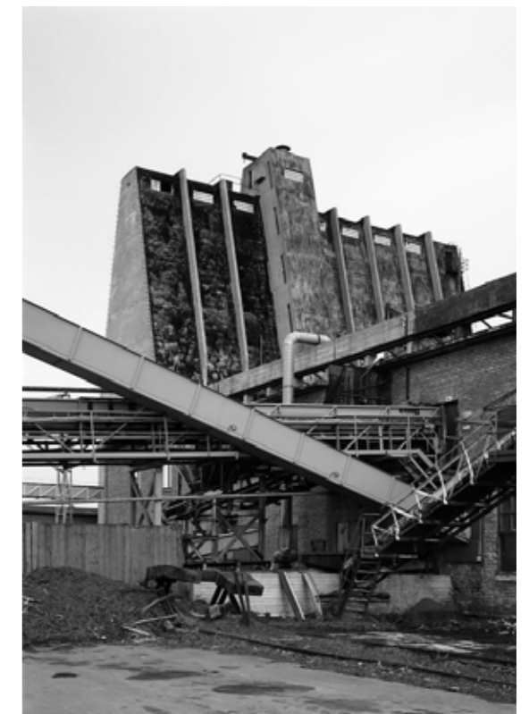
AaltoSiilo, 1980s, shortly after the closure of the Toppila Pulp Mill. Photograph by Raimo Ahonen
