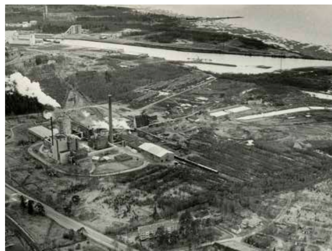
Aerial photo of the Toppila Ltd Factory in 1985. Kaleva archives
