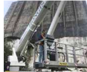
Renovation works begin: cleaning the Silo
