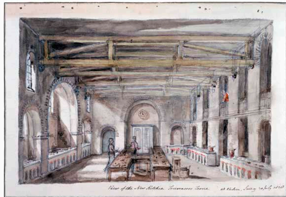
Plate 23: (SM 52/5/44) View of proposed kitchen. Soane designed this dramatic new double height kitchen to sit directly below the New Temple. Its great width necessitated the use of trussed timber girders to carry the floor of the Temple above.
