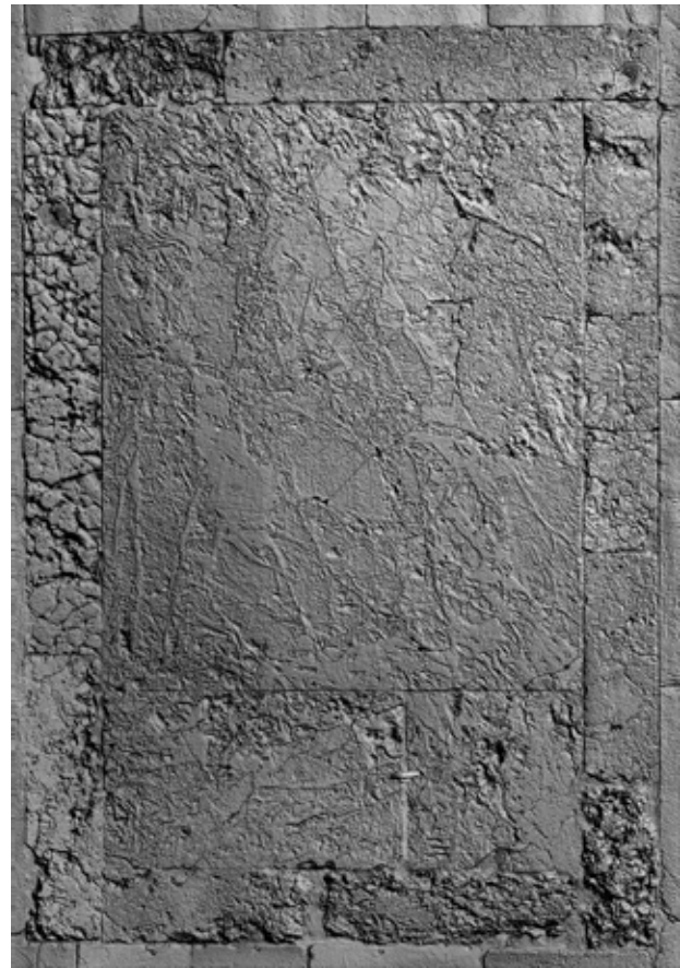
9 Factum Foundation's 3D render from the surface recording of the marble cladding from the west exterior wall of the Treasury of San Marco, Venice
