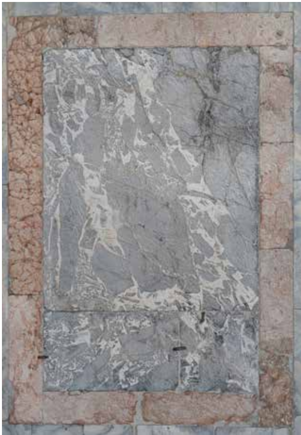
8 Factum Foundation's 3D render of the color and relief information merged of the marble cladding from the west exterior wall of the Treasury of San Marco, Venice
