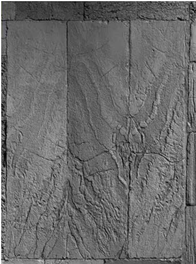
4 Factum Foundation's 3D render from the surface recording of the marble cladding from the west exterior wall of the Treasury of San Marco, Venice
