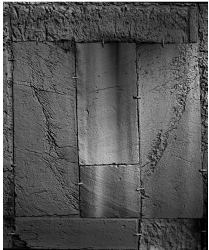
11 Factum Foundation's 3D render from the surface recording of the marble cladding from the south exterior wall of the Treasury of San Marco, Venice
