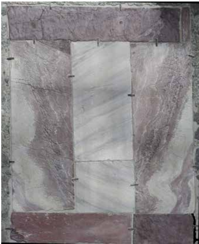
10 Factum Foundation's color 3D render of the color and relief information merged of the marble cladding from the south exterior wall of the Treasury of San Marco, Venice
