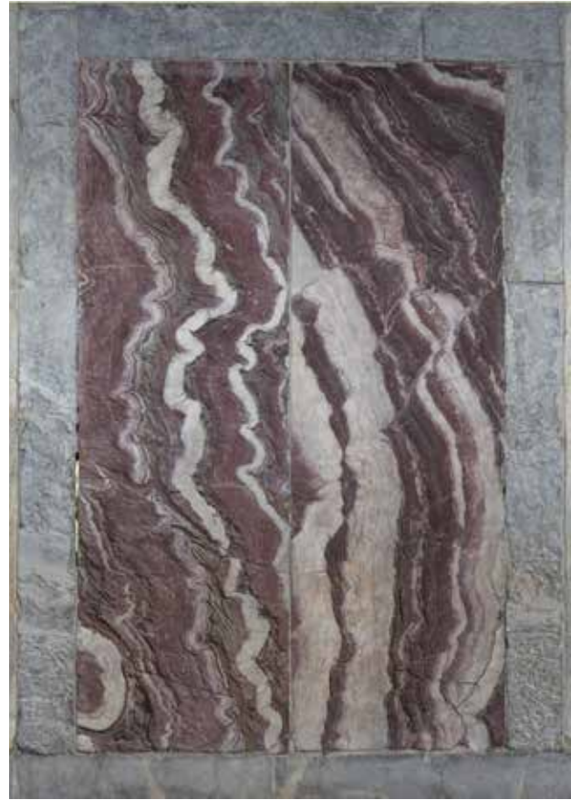
7 Factum Foundation's 3D render of the color and relief information merged of the marble cladding from the west exterior wall of the Treasury of San Marco, Venice
