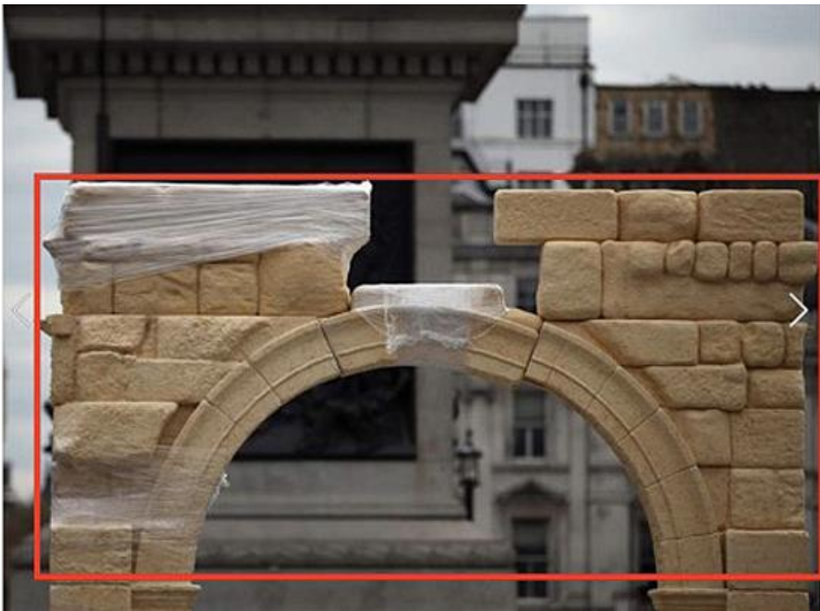
The back of the IDA copy. Note the uniformity of colour and texture; the bricks all fused together and smoothed, looking like bars of soap. Many of the specific details do not correspond to the original central arch.
