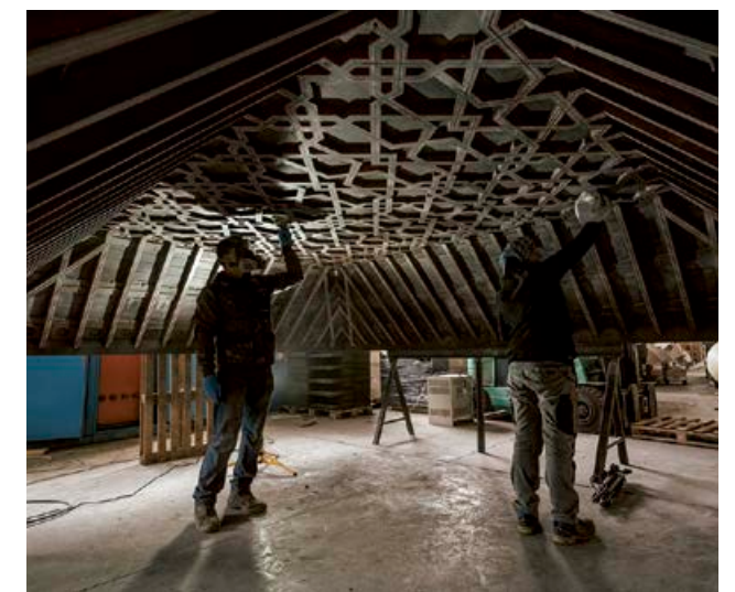
The ceiling of Room B is a tribute to traditional style mudéjar timber ceilings from 16th-17th-century. The installation was designed to incorporate the existing timber trusses of the original roof structure in the exhibition space.
