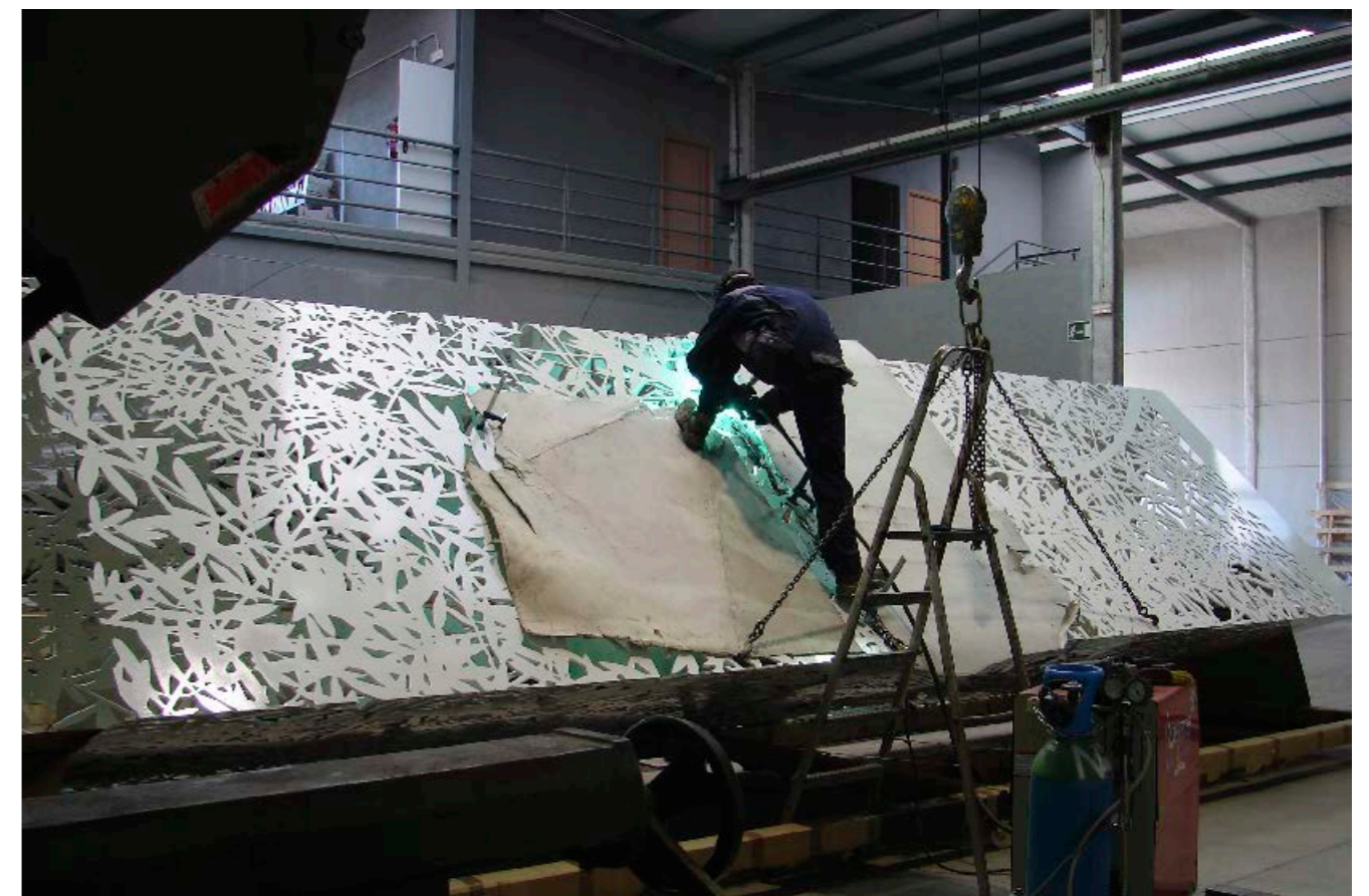
Welding stainless steel
