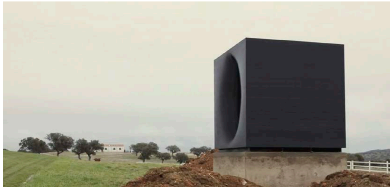
Installed in Ciudad Real, Spain
