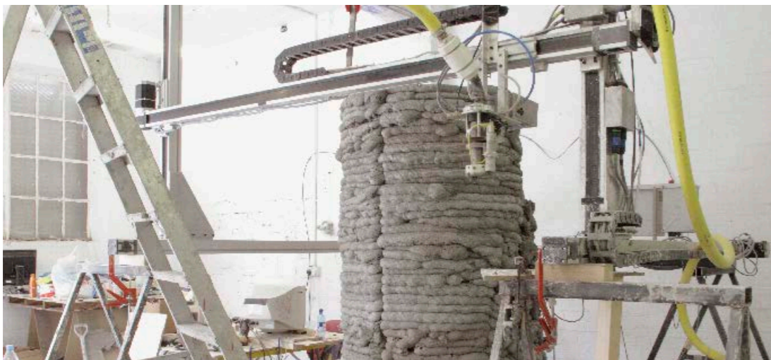
The second concrete printer working in ANISH KAPOOR's studio
