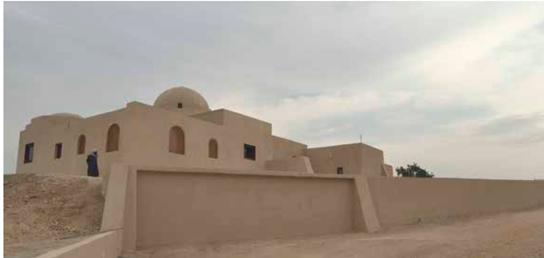
Stoppelaere House after restoration by Tarek Waly and the local team.
